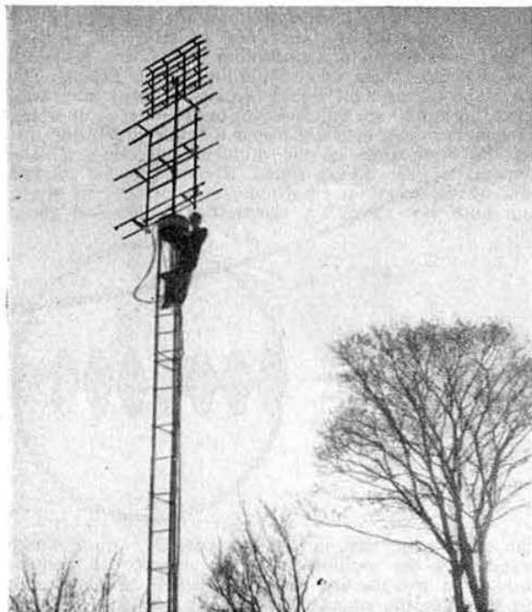
A view of the aerial system at G2DUS/T, Wallington near Baldock, Herts. The home-made 40 ft tower supports a 12 ft rotatable head which carries a 32 element array for 70 cm and a 12 element 2m beam.
